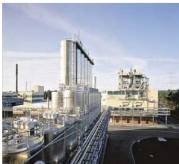
In the petrochemical industry, ZSB busbar applies widely
